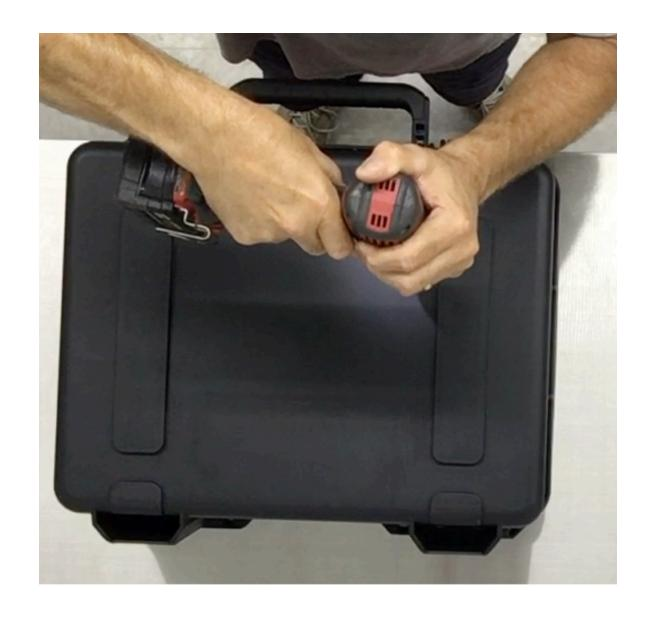
**Step 8** Remove the Slider plate from the case. Use the 21/64" drill bit and electric drill to enlarge the  $\frac{1}{4}$ " pilot hole.
