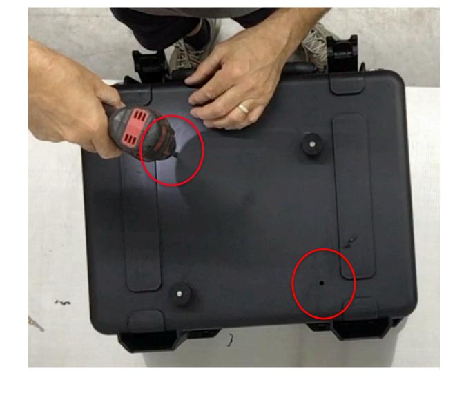
**Step 14** Remove the Slider rack and pucks from the case. Use the 21/64" drill bit and electric drill to enlarge the last 2 1/4" pilot holes.
